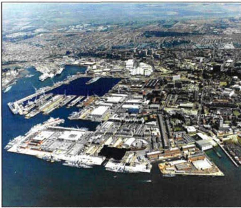
● New jetties have been built along the western edge of Portsmouth Naval Base
