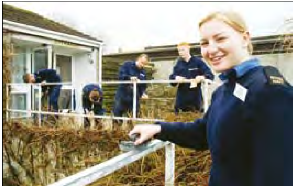
● Trainee Engineering Technician Brooke Wilson and her fellow trainees rub down the paintwork ready for repainting at Pengover Residential Home
