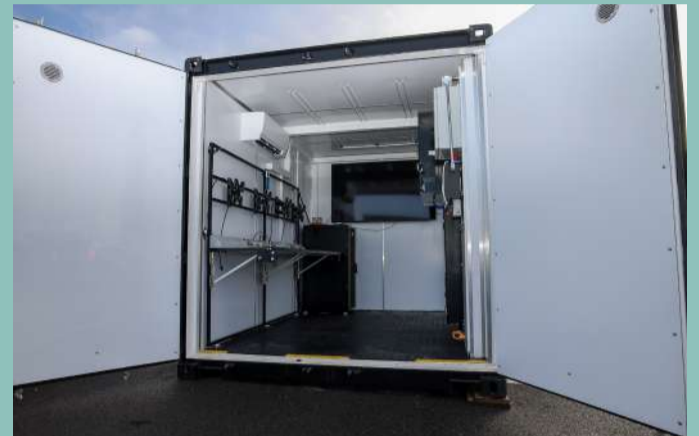
A POD fitted with IT equipment
